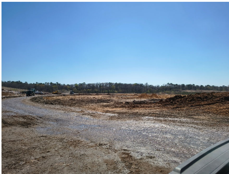
Looking south over Cell 5 active area
