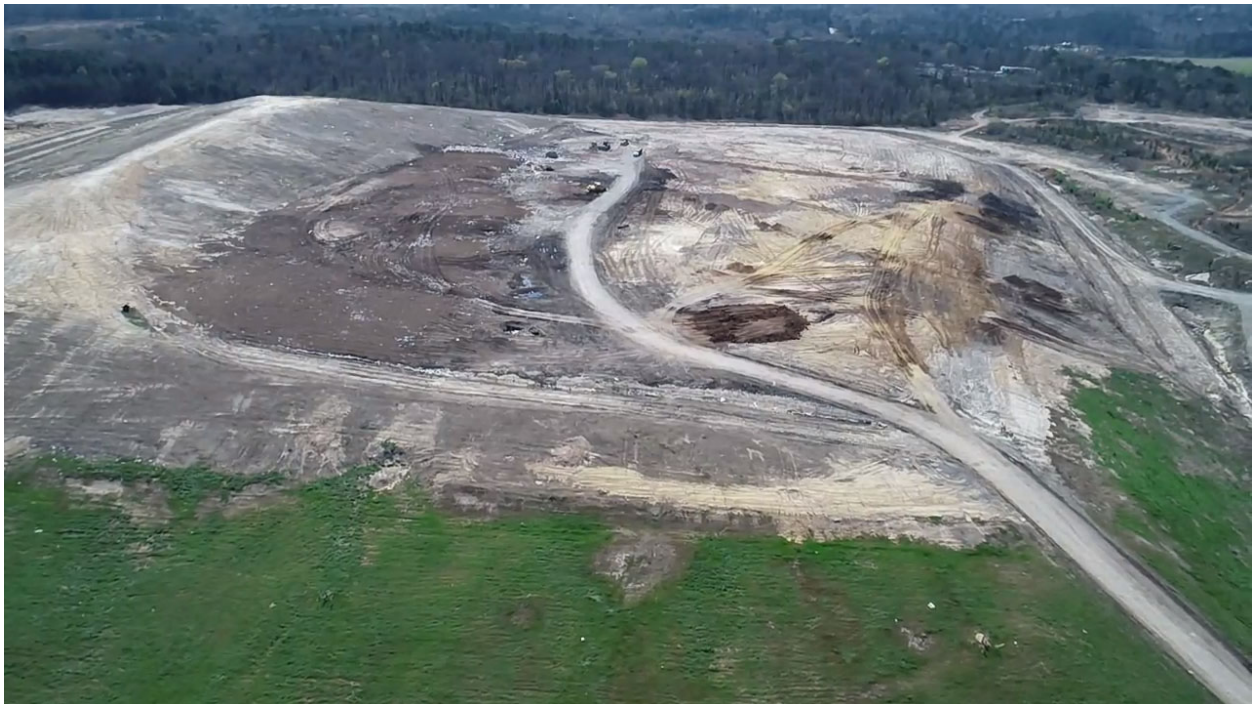
Looking S over Cell 5 (Active area)
